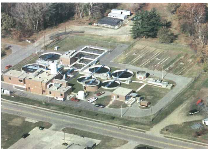
City of Hastings Treatment Plant
